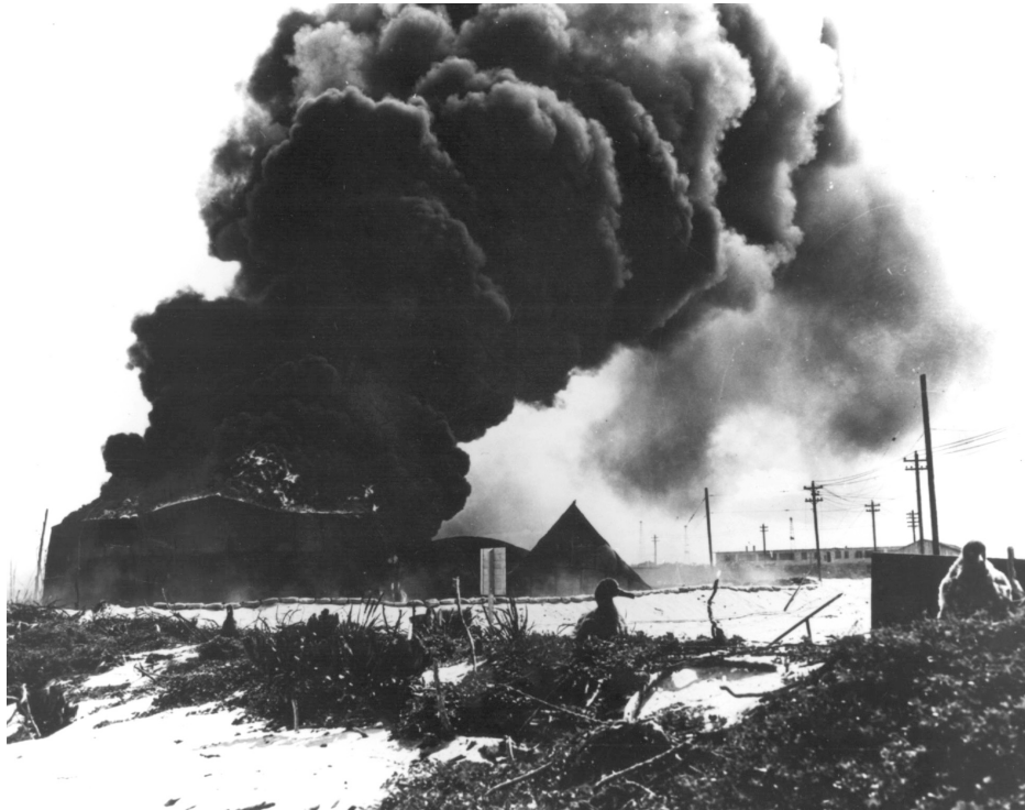
Although the initial strike on Midway caused heavy damage, as seen here on Sand Island, a second strike was needed.
